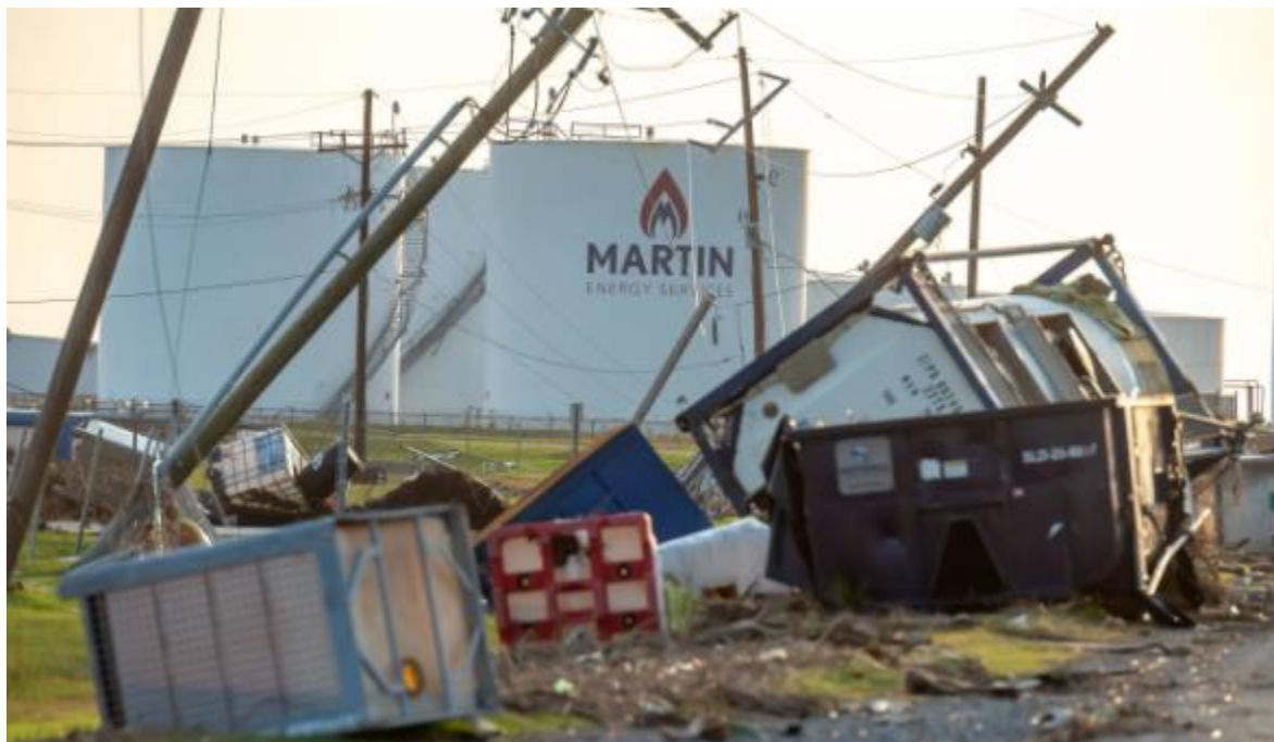
Image 5. Hurricane Ida destruction at Port Fourchon, shown Thursday, Sept. 2, 2021, four days after the Category 4 storm made landfall there. Photo Scott Clause/Lafayette Daily Advertiser
